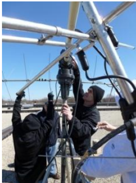
Assembling the Az-El antenna rotor
