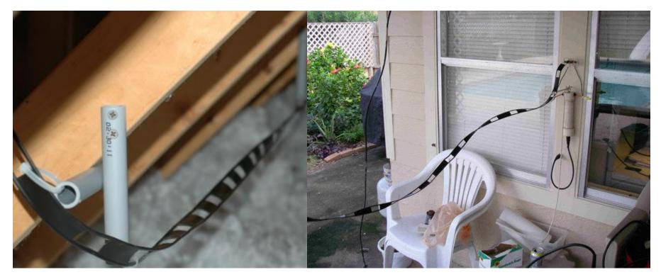
Ladder Line should be installed away from objects
