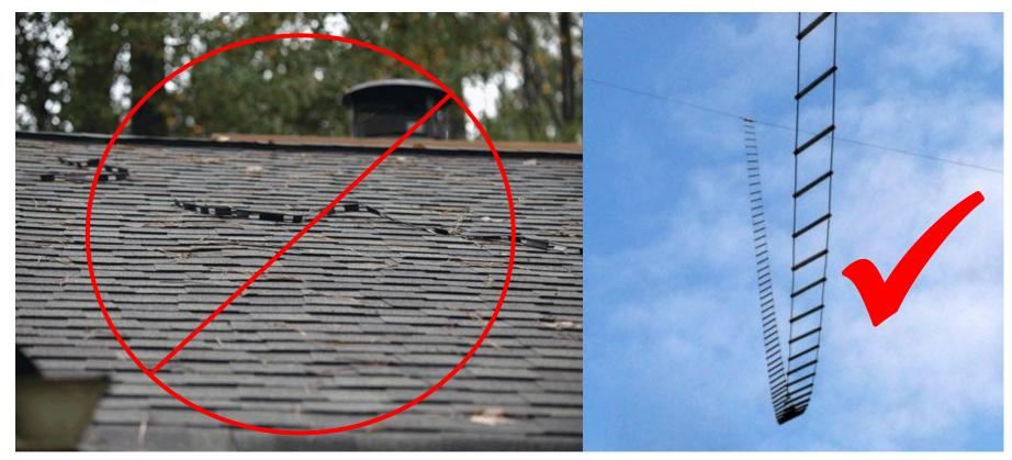
Ladder Line should be installed away from objects
