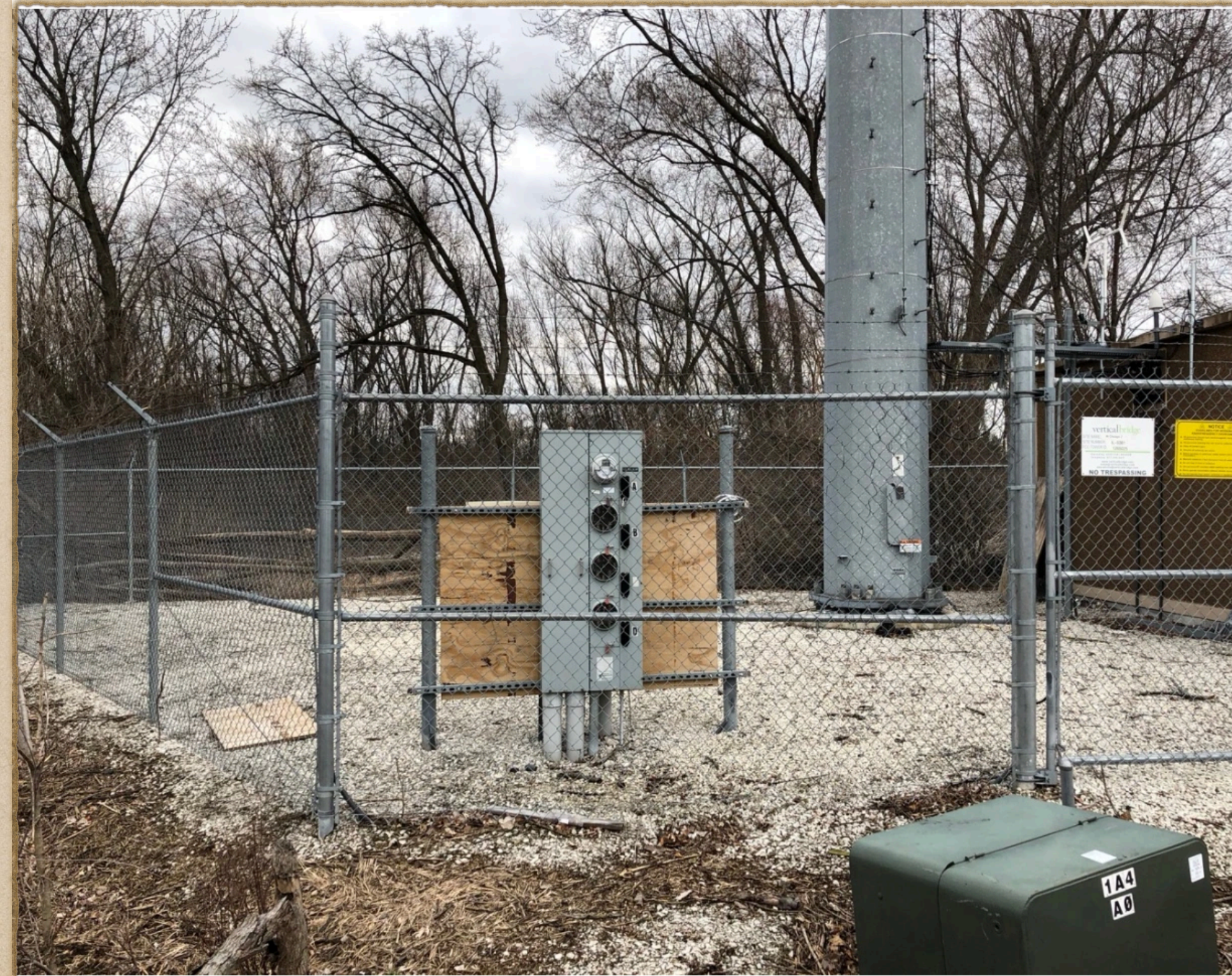
The tower base and perimeter fence.
