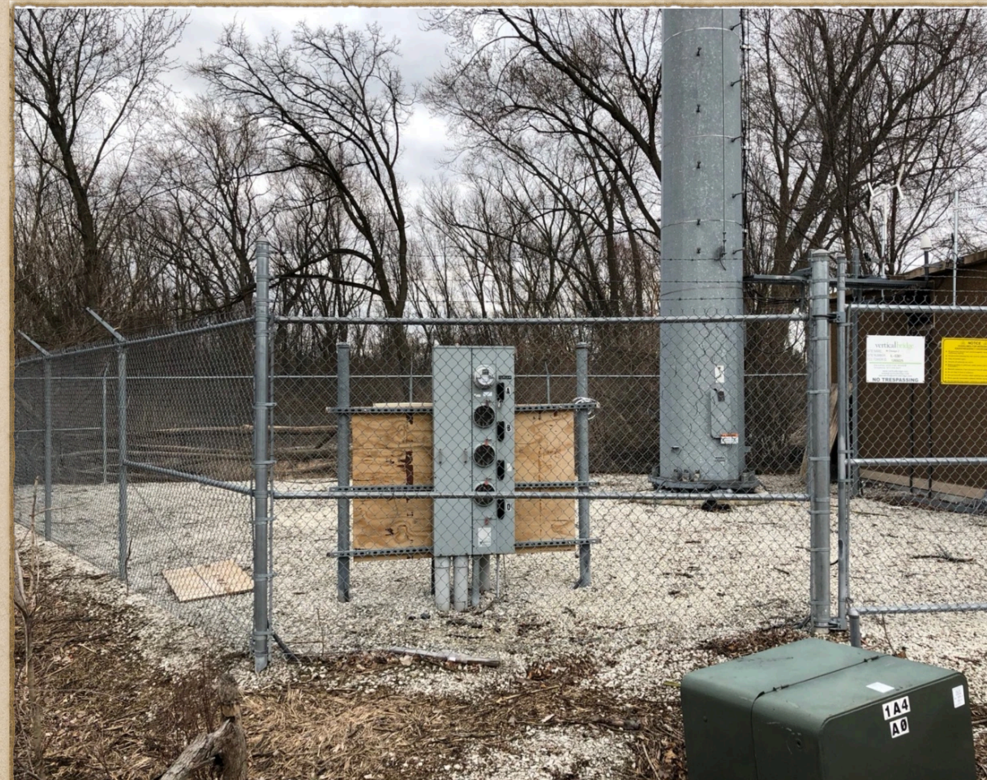
The tower base and perimeter fence.
